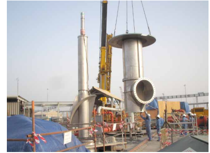
Installation of cooling water pump
