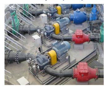
This project is to upgrade five distribution pumping stations in Doha feeding the potable water to in the most of Doha city. The potable water is transmitted from Ras Laffan Desalination Plant at the north of Qatar. Torishima supplied and installed all Electrical, Mechanical and Instrument / Control System.
