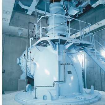
Dewatering pump with adjustable vane (Size:2400mm, Driver:1103kW)
