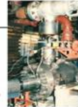
Barrel type B.F.P. (Dalian Power Station)
