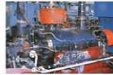
Barrel type B.F.P. (Auraya Power Station)
