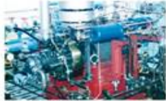
Barrel type B.F.P. (Jandar Power Plant)
